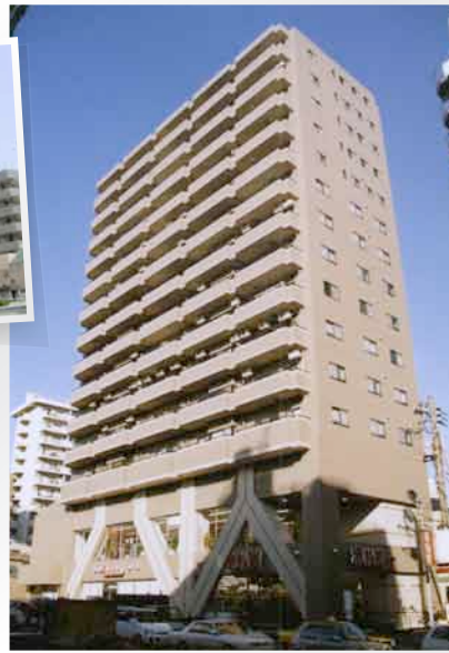
High City Kyosumi used 1500mm diameter isolators that were the largest isolators ever built.
