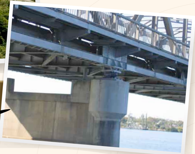
Rio Vista Bridge Typical location of an isolator in the retrofitted Rio Vista Bridge in California
