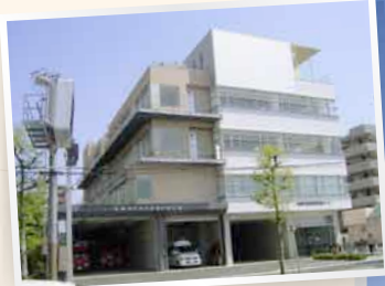
The Funabashi Fire Station is one of many fire stations in Japan that are base isolated.
