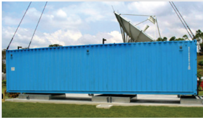
A self-contained data center being installed in Costa Rica.
